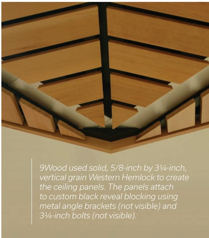
9Wood used solid, 5/8-inch by 3¼-inch, vertical grain Western Hemlock to create the ceiling panels. The panels attach to custom black reveal blocking using metal angle brackets (not visible) and 3¼-inch bolts (not visible).
