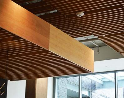
The wood grille ceiling has solid, clear Western Hemlock wood members with flat grain on the primary faces and vertical grain on the secondary faces. Matching fascia trims are veneer on fire-rated substrate.
