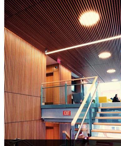
The 18,075 sq. ft. of wood grille ceilings are found on multiple levels. They line up with the wall systems installed by a millwork contractor.
