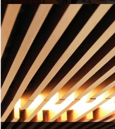
9Wood designed and fabricated 72 special wood grille access panels to cover two kinds of circular light fixtures in the space. The access panels float seamlessly overhead.
