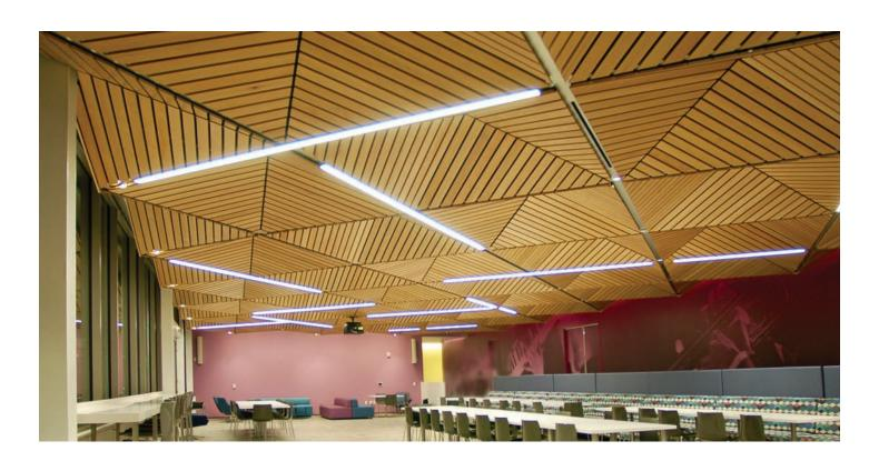
STUDIOS Architecture, San Francisco, Calif., wanted a "folded triangular acoustical wood ceiling." In response, 9Wood created a linear wood ceiling system of "pyramids and inverse pyramids."
