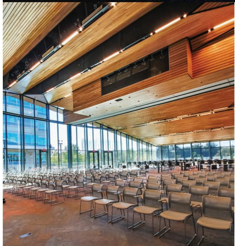
The multipurpose room showcases ceiling bays set at angles. The ceiling bays or "troughs" house sprinkler heads, lighting and air diffusers.
