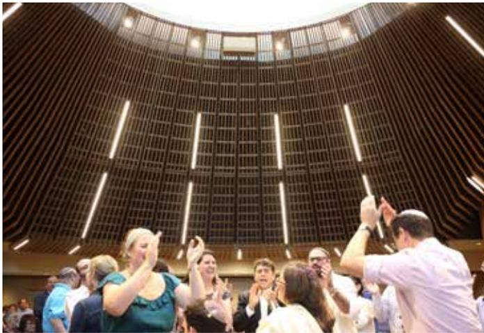
*The spacing between wood grille slats gets narrower – from a 1' separation between slats and finishing at 2" between them – as the ceiling curves upward.*
