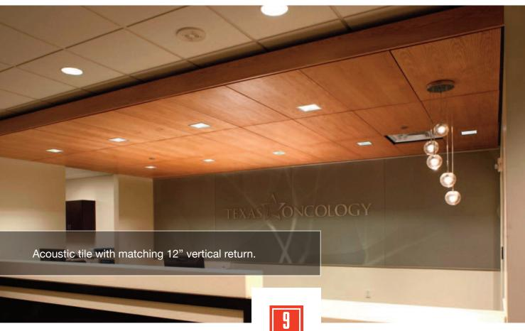
offered accessibility by allowing the individual panels to be removed after installation, while the XL Channel system was ideal for the fixed panels around light fixtures. However, because the two attachment systems yielded different installed depths, a new fitting was developed specifically for this project, to re-align the faces of the panels.
