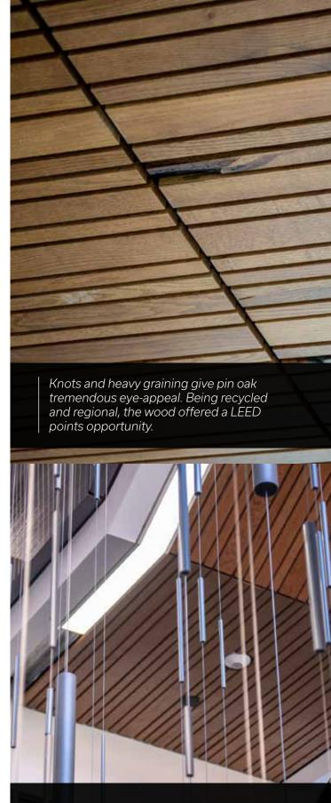
Elements of a hanging sculpture were tuned to the acoustical properties of the wood ceilings. "The sculptor turned our panels into a sound resonance system," Bohl says. The installer had to make many cuts to transition the linear ceilings around the varying pitches and staircase elevations.
