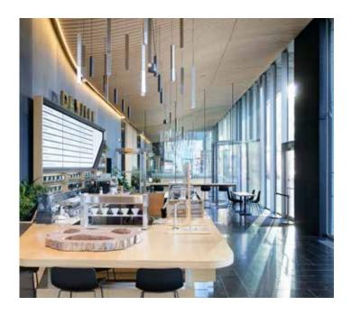
The wood grille ceilings flow as a compound wave in the coffee shop. 9Wood used a GPS point cloud of the space to build a 36' by 8' mockup of the ceiling before its installation.
