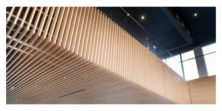
The monolithic wood grille ceilings create horizontal and vertical surfaces that line up perfectly. The general contractor's surveying team plotted the lobby's GPS points, creating a point cloud that enabled 9Wood to produce cross piece grille panels that line up and seem to float in the space.
