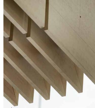
3D modeling of the ceiling design contributed to a precise ceiling installation. "The product lined up so easily it wasn't necessary to do any rework," says Aaron Macdonald, project manager at ICON West Construction.
