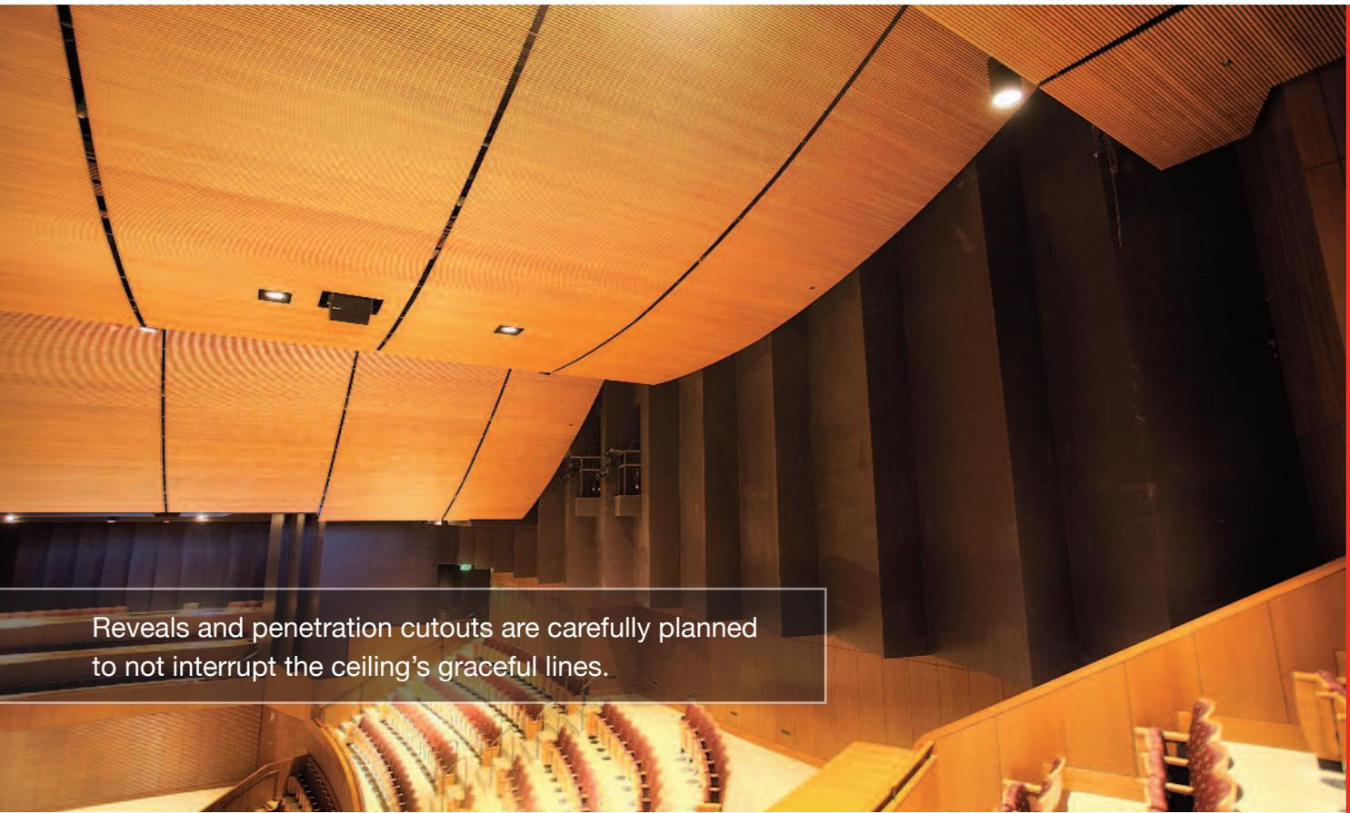
Reveals and penetration cutouts are carefully planned to not interrupt the ceiling's graceful lines.
