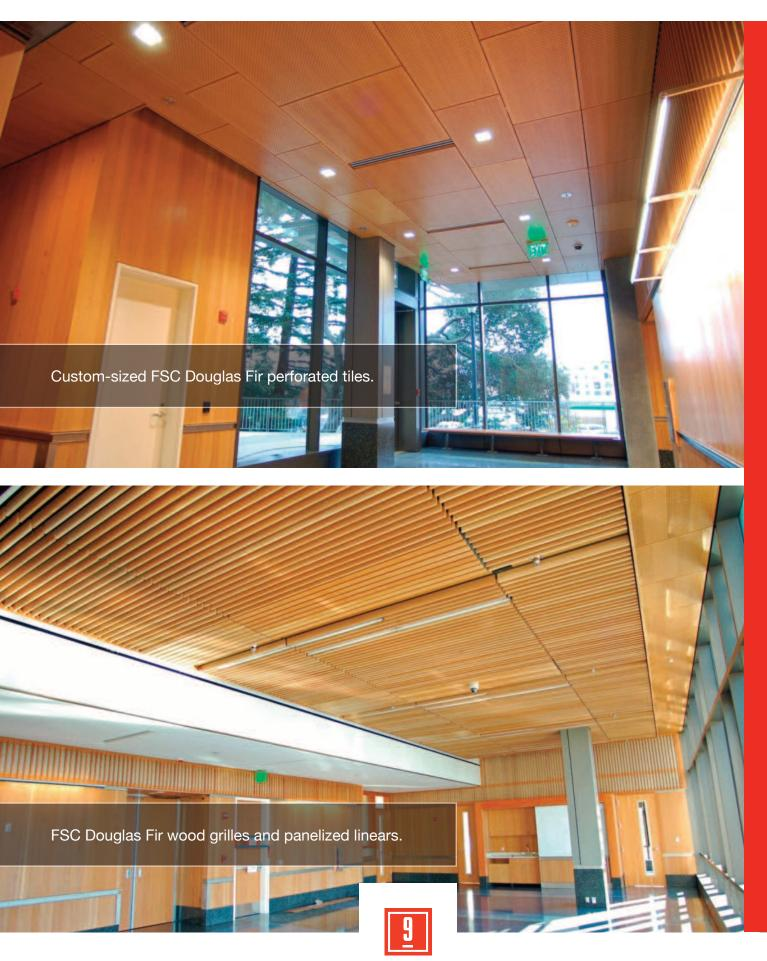
9Wood Lift & Lock attachment that required a standard grid configuration, Ratzlaff coordinated with Lindner of Germany to devise a custom suspension that would more easily accommodate the custom, angled perimeters. This system was the definition of integration: 9Wood and Lindner working together.
