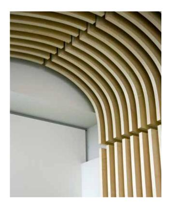
9Wood produced wall and ceiling grilles that lined up without knowing the geometry of the suspension, which was decided upon in the field.
