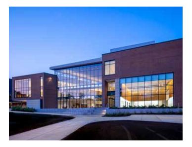
The Minskoff Pavilion features a steel frame with composite concrete decks, brick veneer walls and wood slat ceilings and walls.
