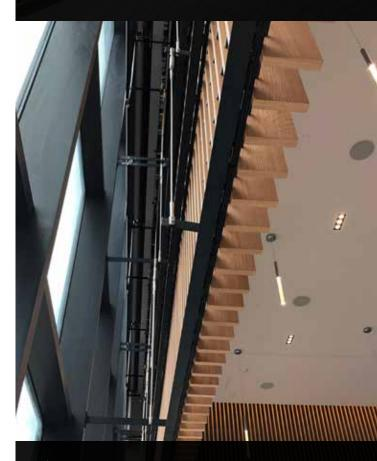
Mod Interiors, along with the design team, developed an attachment system to suspend the wood grille panels ¼" in front of blackout window shades in the multipurpose room.
