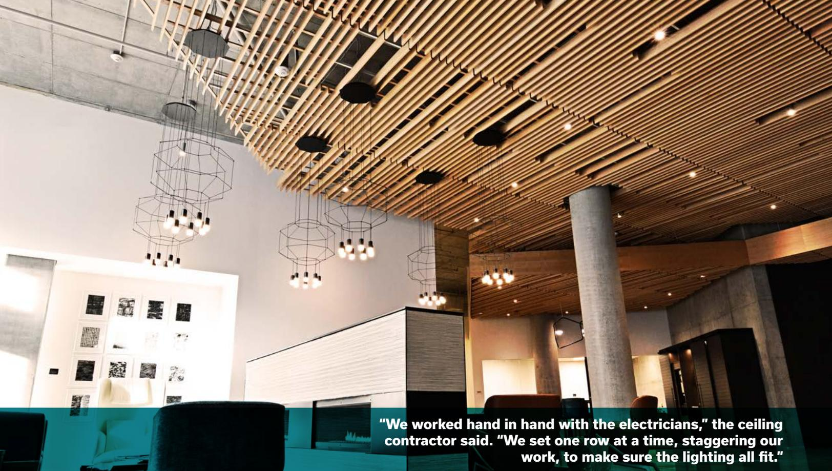
**"We worked hand in hand with the electricians," the ceiling contractor said. "We set one row at a time, staggering our work, to make sure the lighting all fit."**
