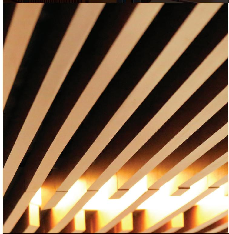
9Wood designed and fabricated 72 special wood grille access panels to cover two kinds of circular light fixtures in the space. The access panels float seamlessly overhead.
