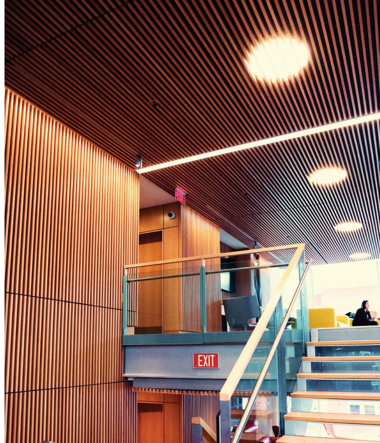
The 18,075 sq. ft. of wood grille ceilings are found on multiple levels. They line up with the wall systems installed by a millwork contractor.
