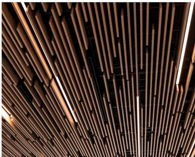
The wood grille panels had 12 to 15 blades of varying depths and spacings. The ceiling contractor installed each panel in proper sequence like a jigsaw puzzle.
