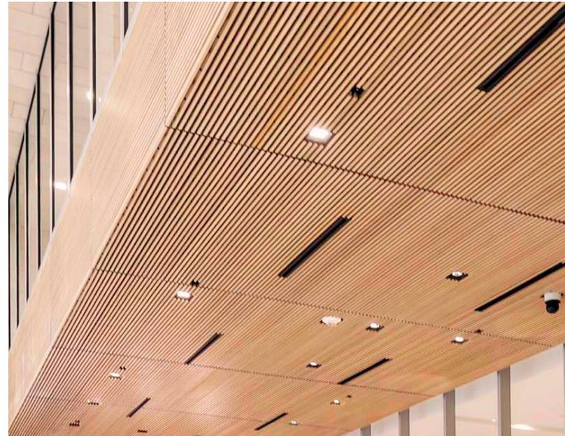
The building features 1,055 wood grille panels that integrate with 106 can lights, 46 slot diffusers, 76 fire sprinklers, 10 fire alarms, and 4 cameras.
